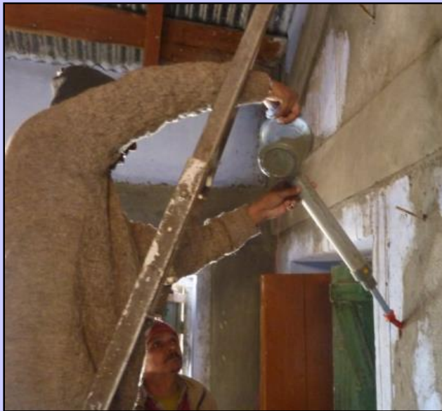
Pump made from plastic pipes and nozzle
