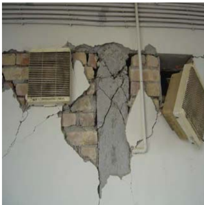
Photo 21: Shear crack in column
