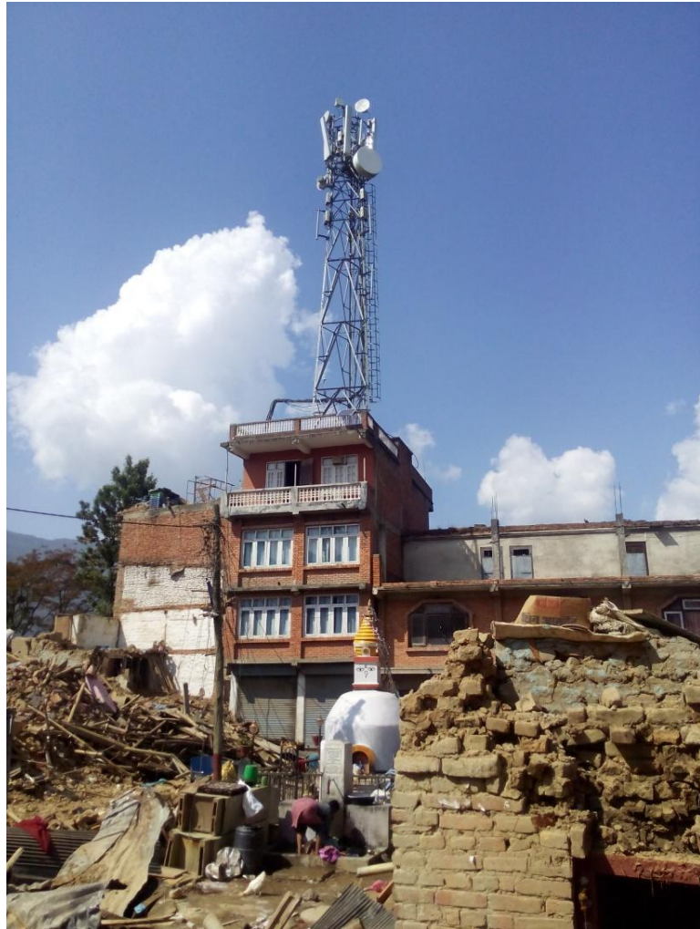
Framed Structure, Dharmasthali (No damage)
