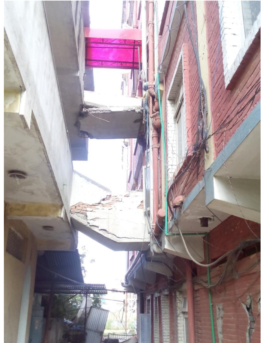
Building Attachment Failures
