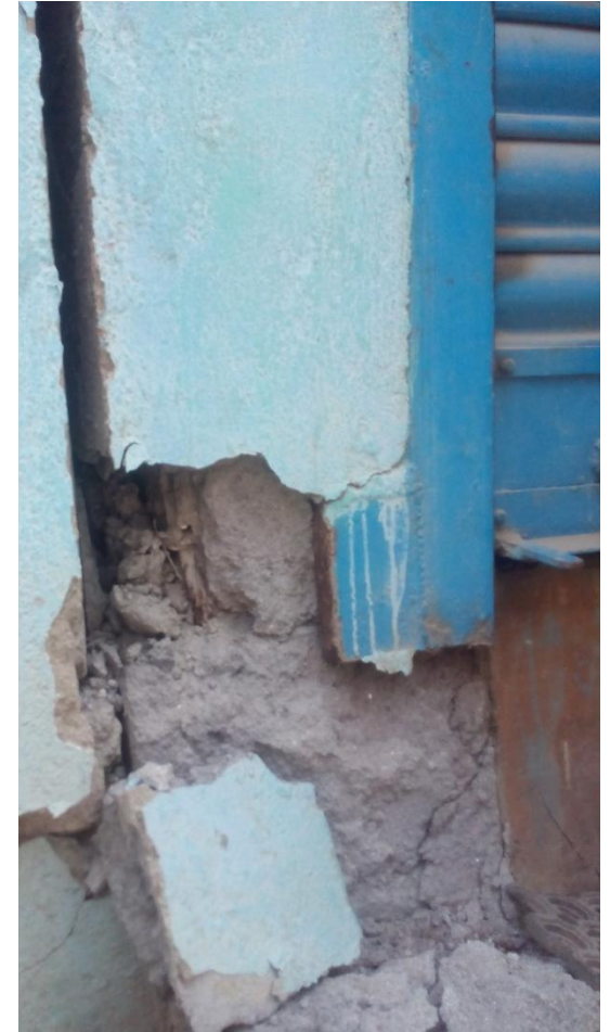
Shutter connection with Column
